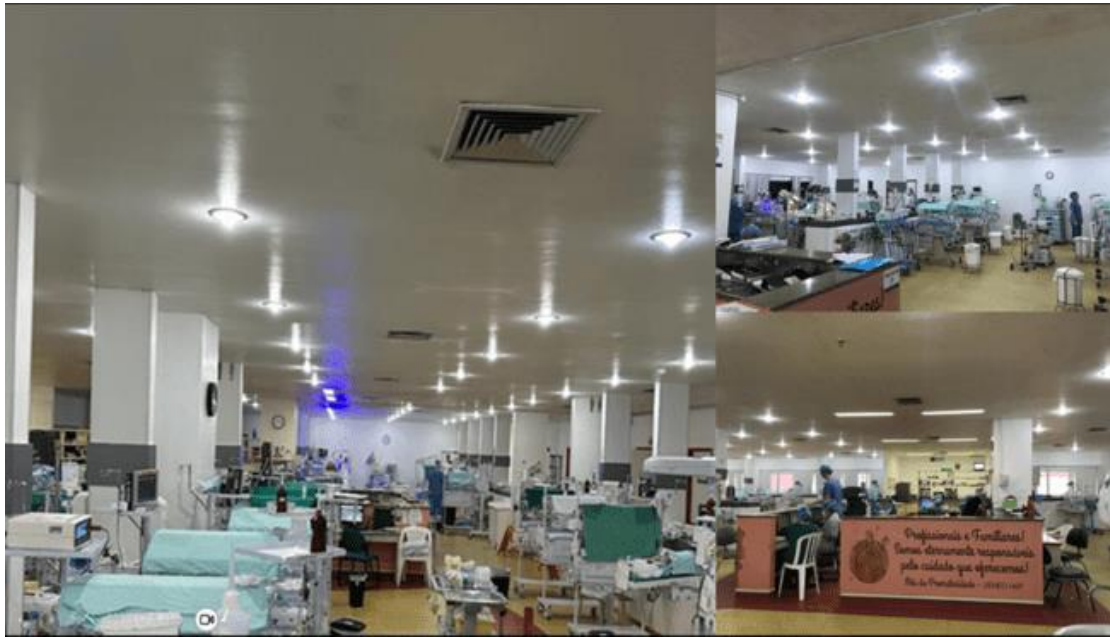
Figura 4 Hospital Geral de Fortaleza (Hospital 2).
