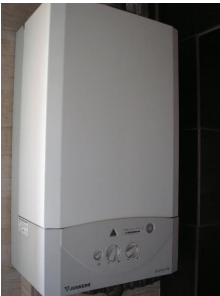
Figura 62 - Caldeira mural a gás natural “Junkers Euroline ZS23-1AE”
