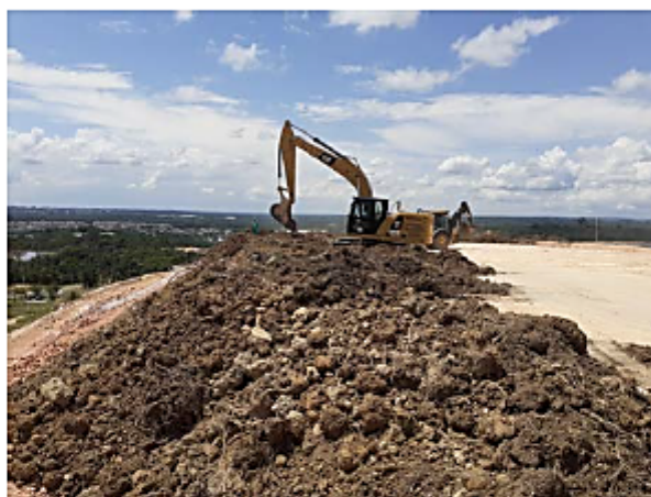
Fig. 2. Backhoe operating in the Manaus public landfill
