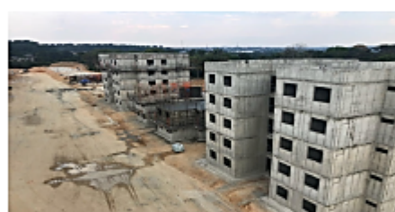
Fig.3: Construction site for residential buildings
