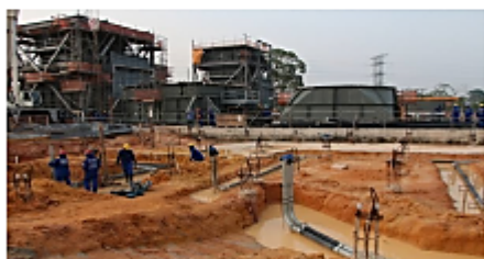
Fig.2: Construction Site of a Thermoelectric Plant
