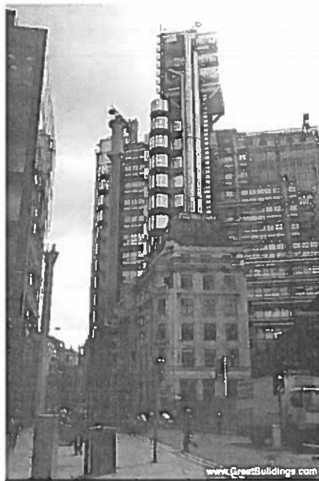
Figura 4.1 – Lloyds Building – Londres ( www.greatbuildings.com )
