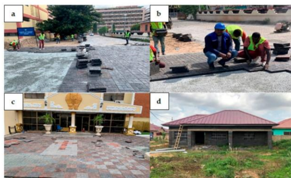
Figure 3. Shredded plastic waste mixed with sand to form pavement blocks. (a) Arranging plastic pavement blocks to lay, (b) plastic pavement blocks being laid, (c) completed laid plastic pavement block, (d) house constructed from plastics. Source: Nelplast Ghana Limited [58].
