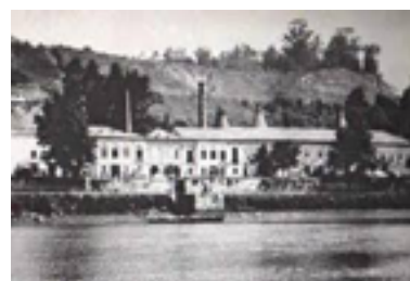
Figura 52, Fábrica de Louça de Massarelos.(2015), Avenida Paiva Couceiro, https://encrypted-tbn3.gstatic.com/images?q=tbn:ANd9GcTNyd5qvICST-qsbt5ryHzspneLubyGZO72QwL-lrg-DBk2UQEe
