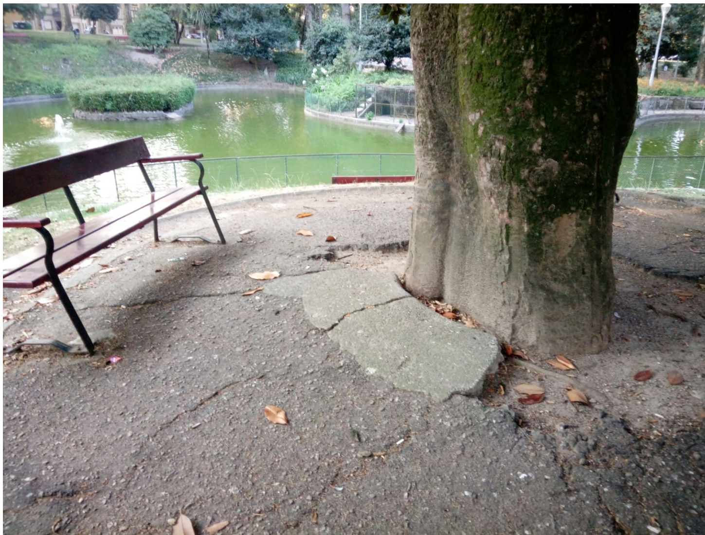
Seat in a terrace at Arca d'Água Garden, Porto.
