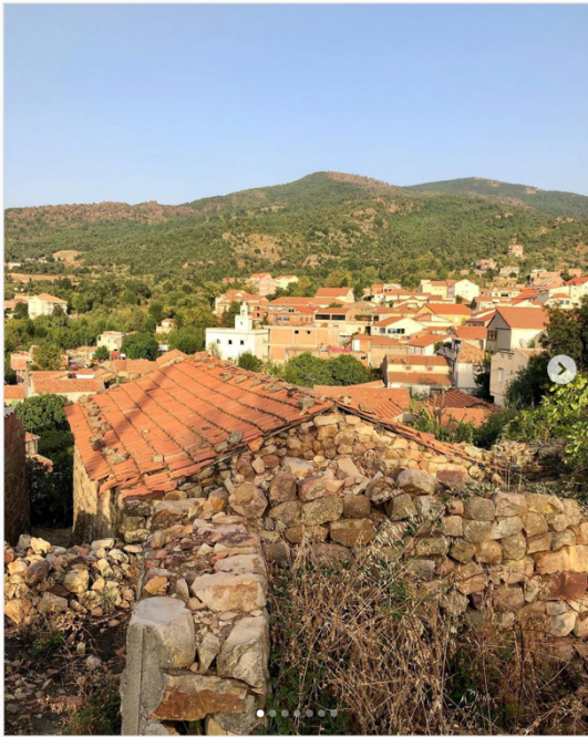
Traditional stone houses in Kabyle villages.
