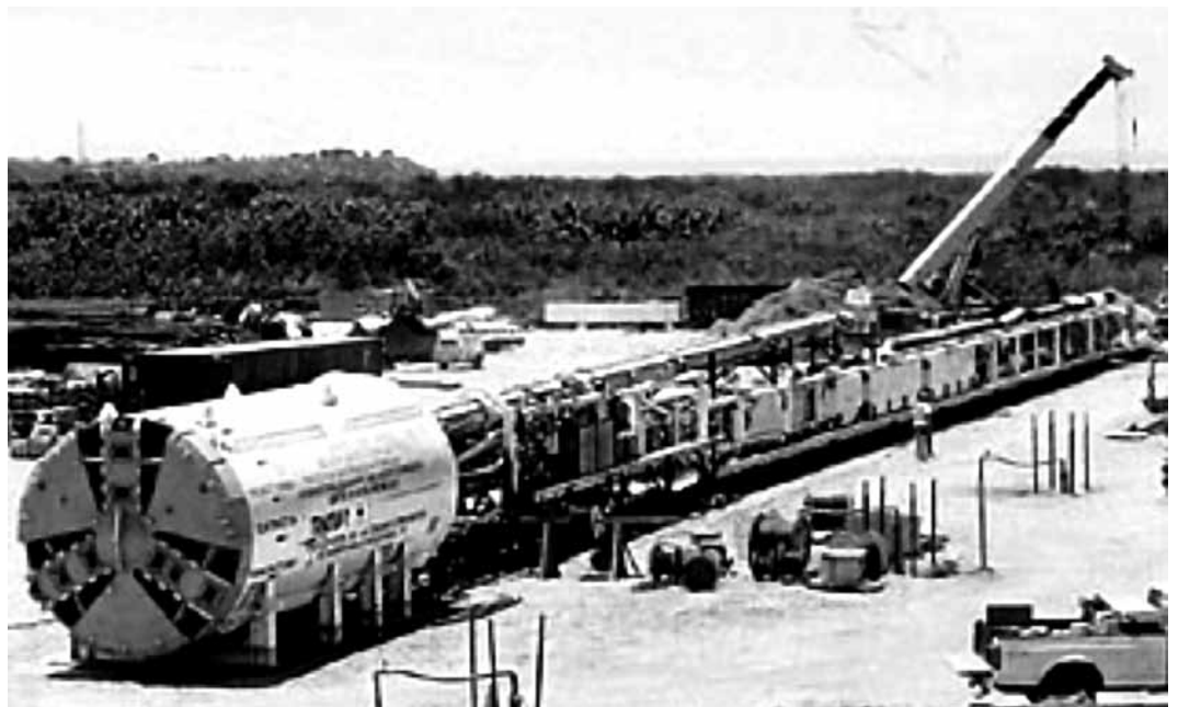
FIGURA 13. TUNELADORA OU TBM ( TUNNEL BORING MACHINE ) (www.msdc.com)
