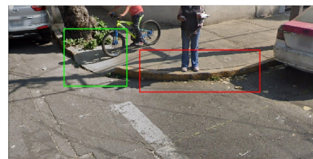
FIGURE 5 | Image with two objects of interest: curb ramp (green) and no curb ramp (red).
